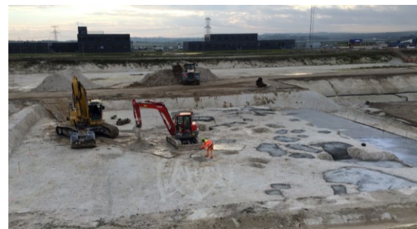
Figure 11: Excavations of 'chimneys'
